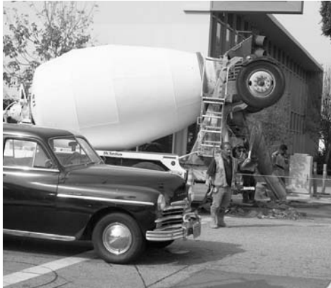
Above: New handicap curbing for Commonwealth/Malden corner.
