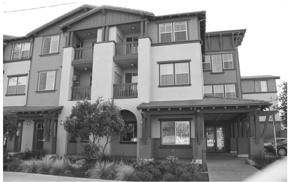
Community of Friends 28-unit Avenida Villas apartments for homeless and mentally ill located in Anaheim. PHOTO BY JERE GREENE
