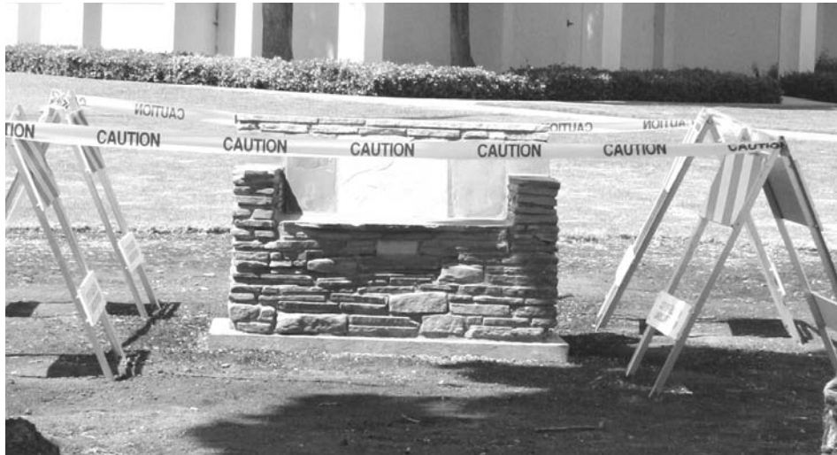
The old sandstone bench at the corner of Commonwealth and Highland in front of City Hall was being crushed by the large Cypress trees so was moved back a bit.
