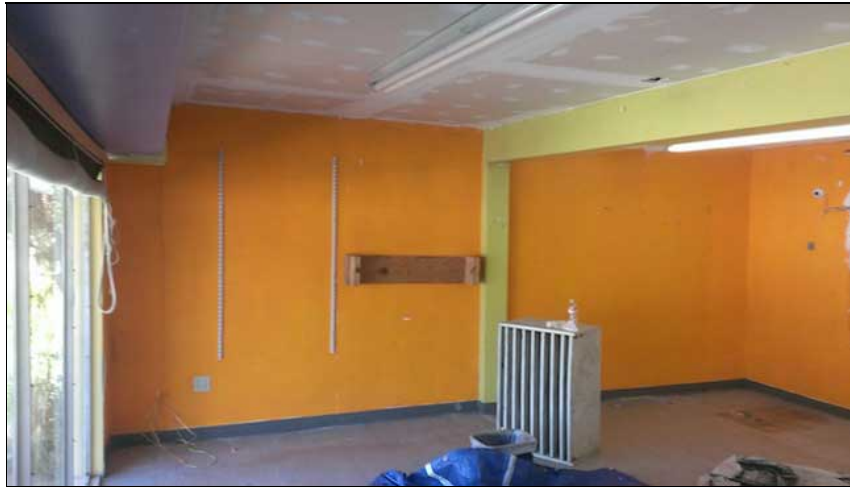
Art classroom renovations in progress
